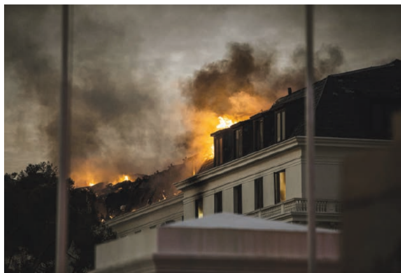
RAGING. Firefighters battle the blaze that engulfed the National Assembly building in Cape Town on 3 January. It is reported the blaze began in the older part of the building. Picture: AFP
