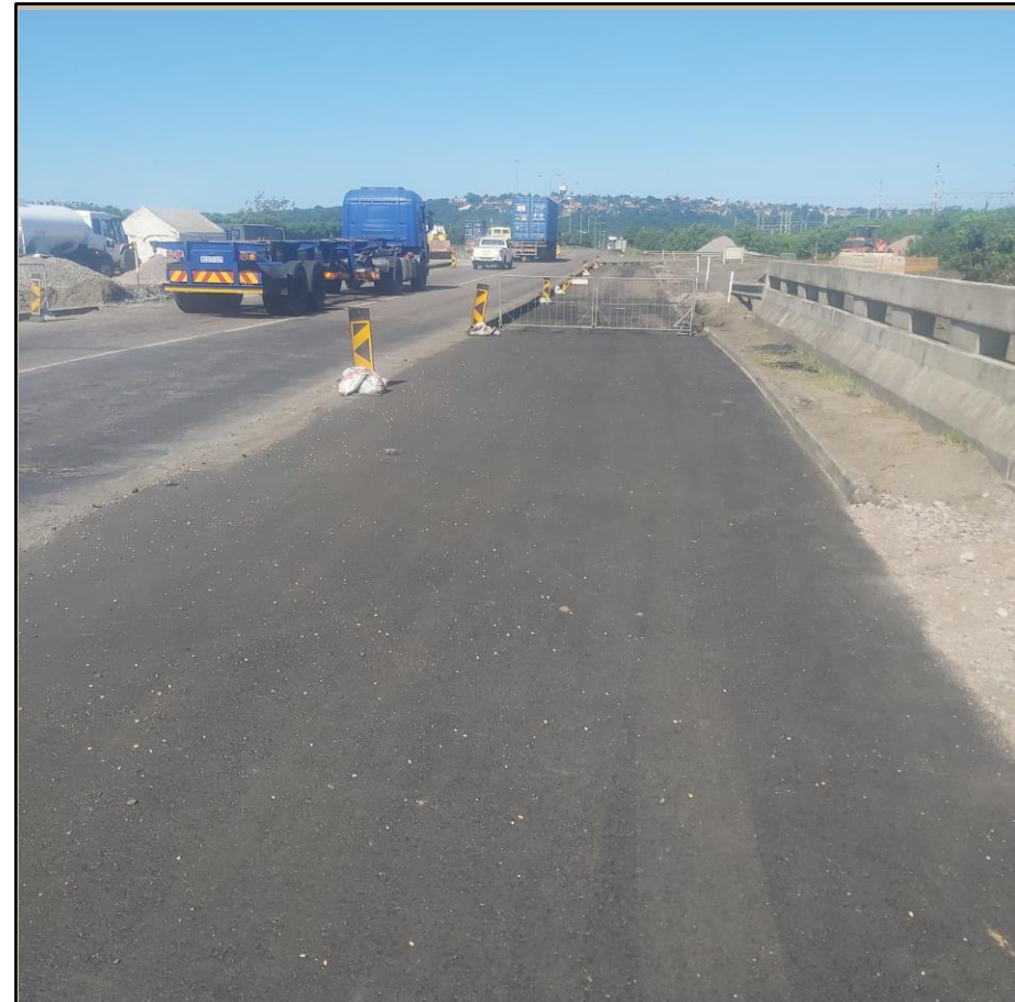
Construction of 3 lane: ~75% complete
