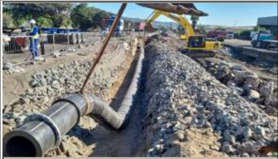
In-bound Lanes: Laying of Sewer Pipes
