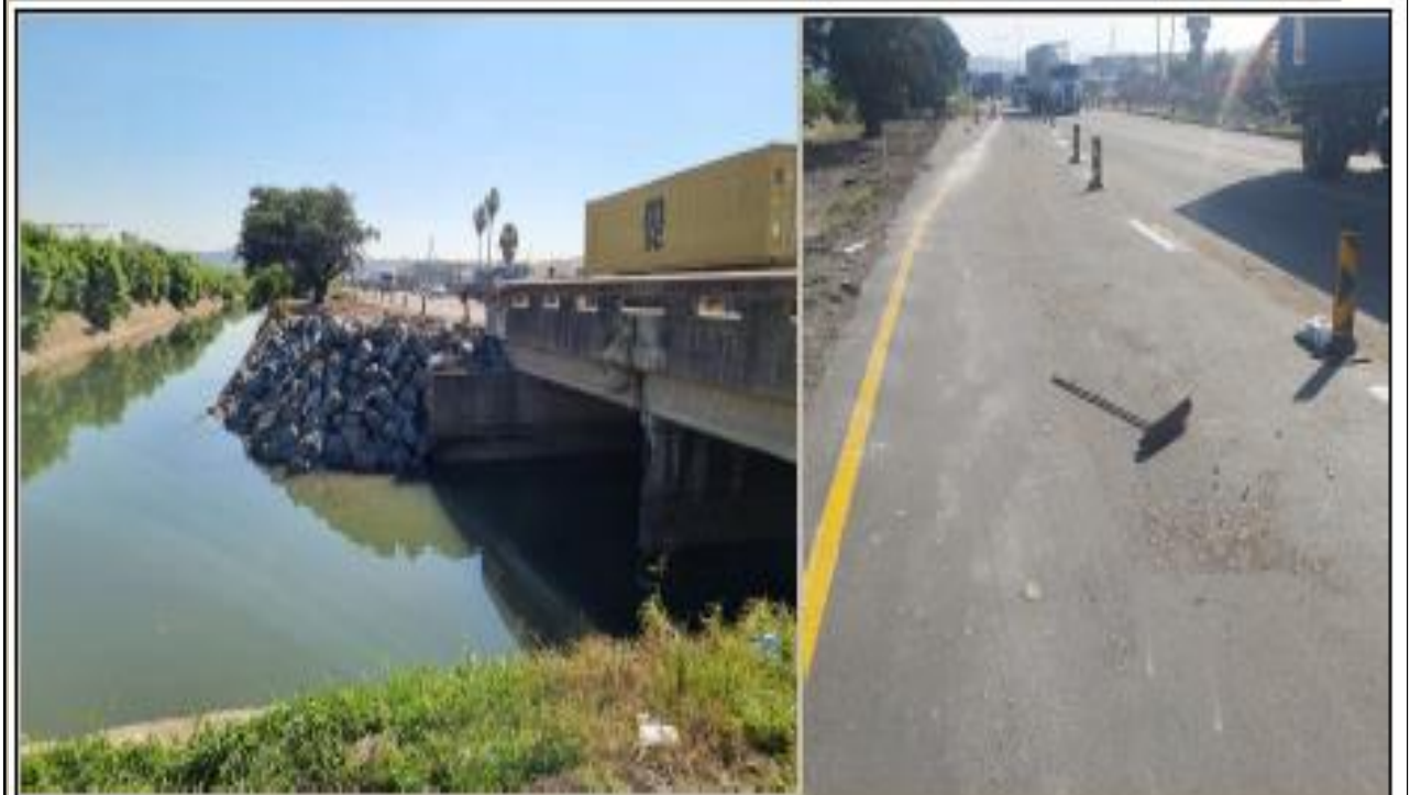
3rd Outbound Lane: Embankment Protection and Cleaning in Readiness for Opening
