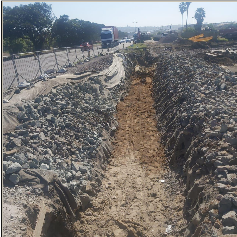
In-bound Lanes: excavation for sewer pipes
